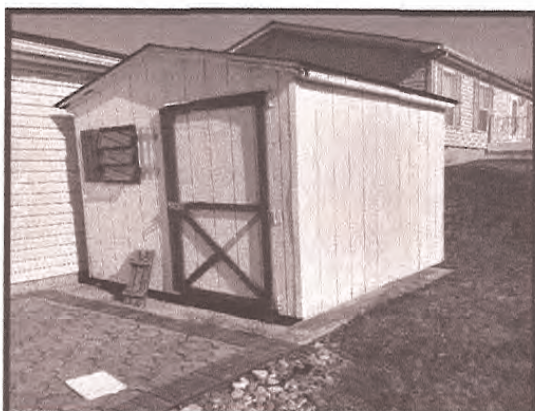
Haven Tree Ct BEFORE.....
