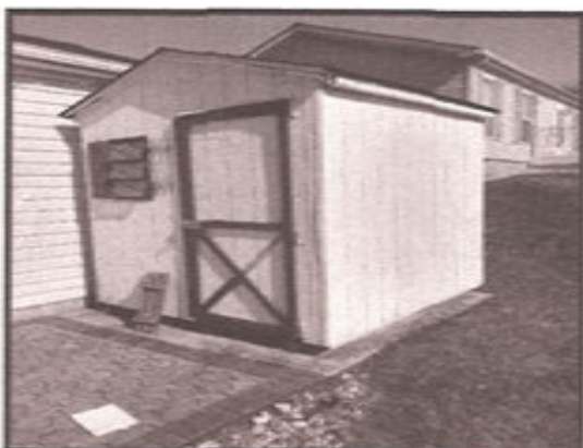
Haven Tree Ct BEFORE.....
