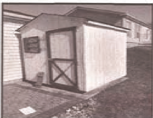
Haven Tree Ct. BEFORE.....
